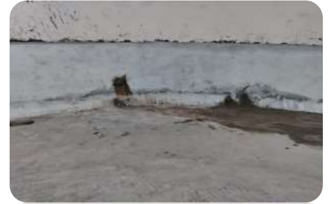
Joints of RCC
