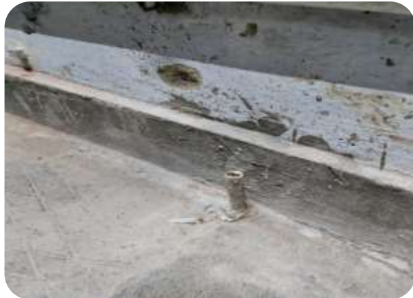
Injection Grouting nipple
