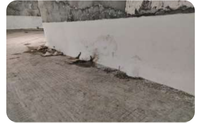
Coating on walls for waterproofing
